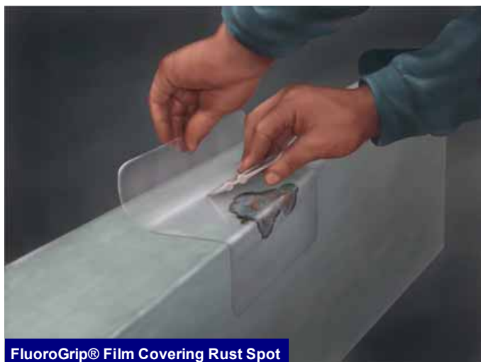
FluoroGrip® Film Covering Rust Spot
